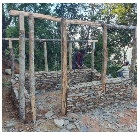
Basic shed being constructed during establishment of a chicken farm
