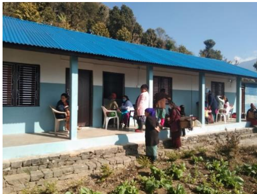
Rebuilt Tawal health post servicing 5 local villages
